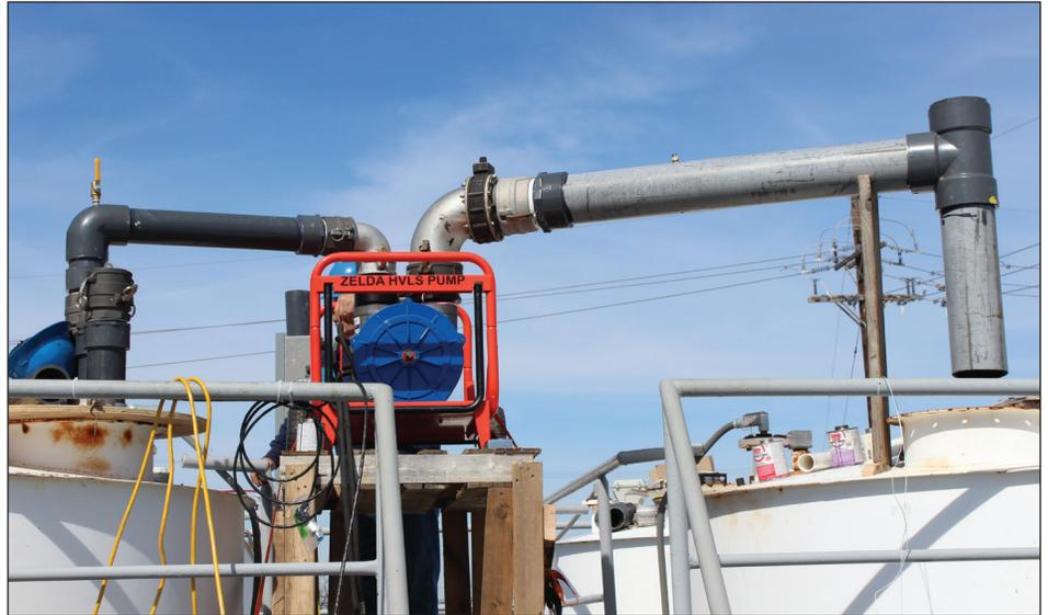
**The Zelda II HVLS pump can be powered by a hydraulic motor or by a hand crank. The low operational speed reduces wear, heat and the possibility of cavitation and emulsification.**
