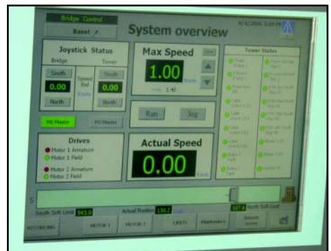
The new bridge drive system includes a computerized system so the tank's bridges may now be controlled and operated from both the control tower and the main bridge.
