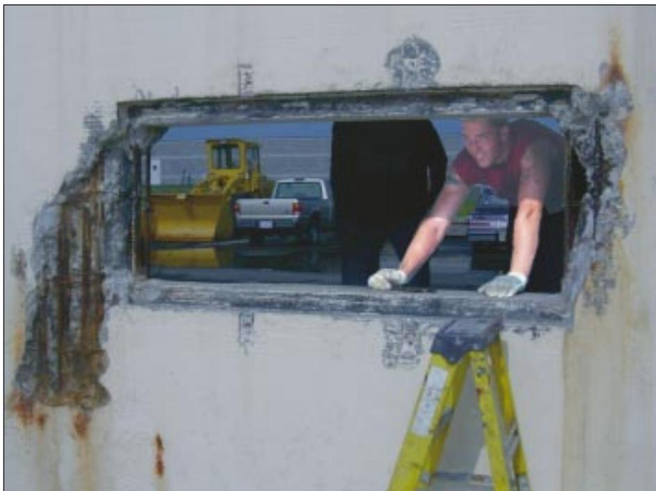
A technician peers through the gaping hole left when the old basin viewing window was removed.
