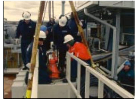
U.S. Coast Guard personnel place a pump into the supply tank.
