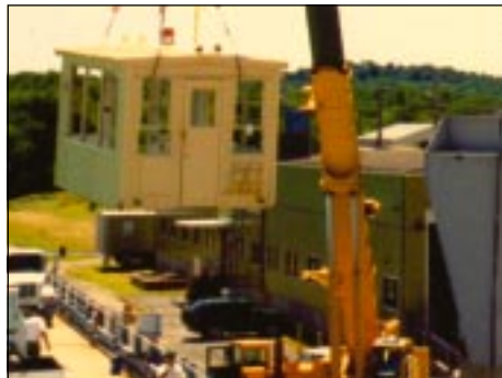
Out with the old bridge house....
