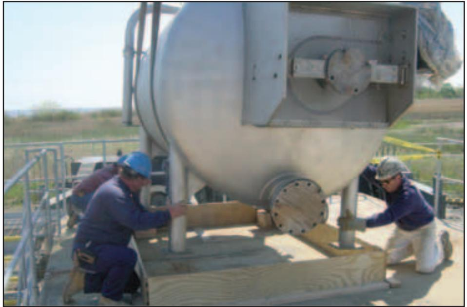
**Construction workers place the new U.S. Filter system onto the concrete filter pad**
