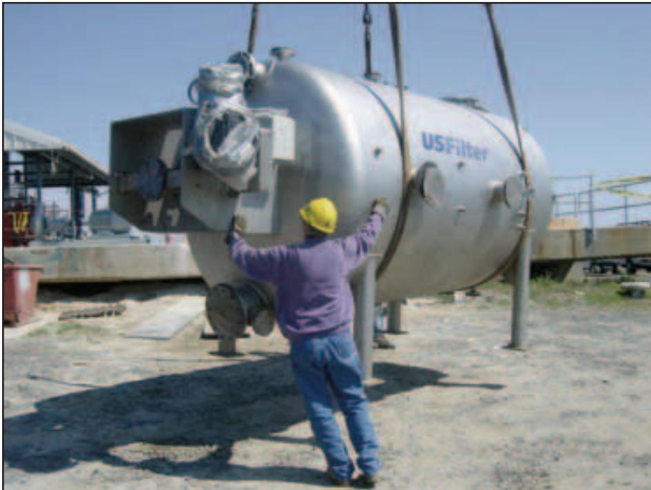
**Construction workers raise new U.S. Filter water filtration unit at the Ohmsett facility**
