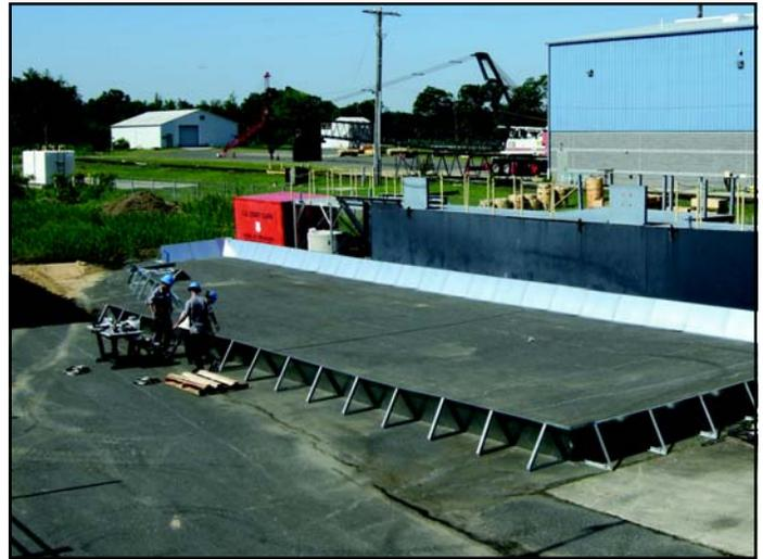
A temporary secondary containment area was constructed where FRAC Tanks were used for test oil storage.
