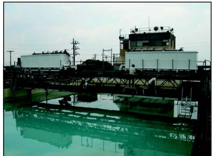
Additional recovery tanks were added to the auxiliary bridge to accommodate the high capacity fluid collection.
