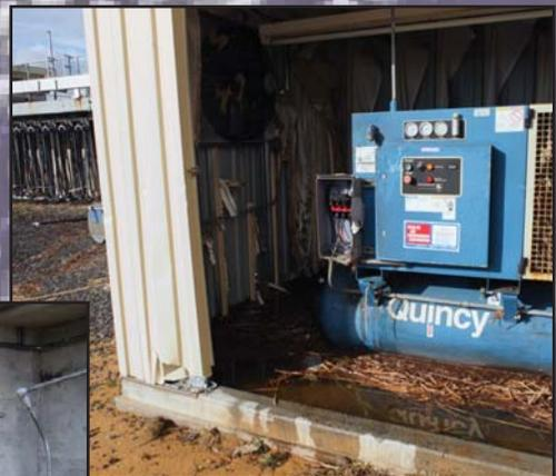
The filter room was underwater and an air compressor was ripped off its mounts during the storm.
