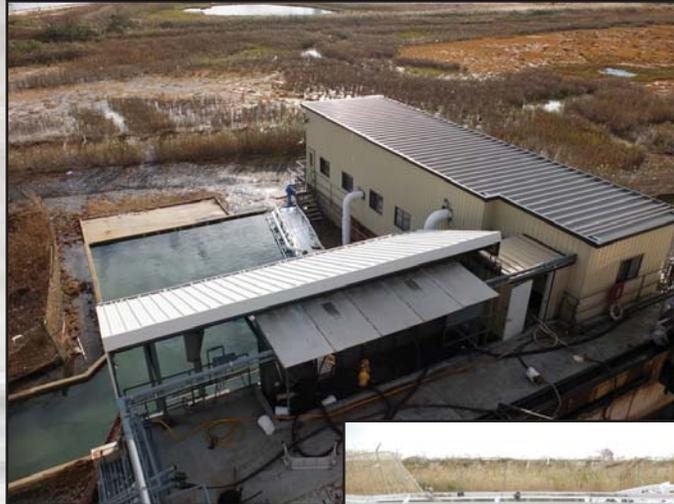
The secondary containment area (Lake Zelman) was flooded due to a crack in a 12-inch filter pipe.
