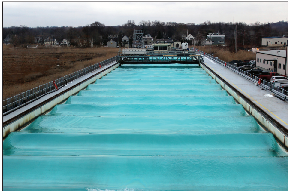
A study of the waves created in the Ohmsett test tank will enable the engineers to create a table which correlates wave height and wavelength with user input settings.
